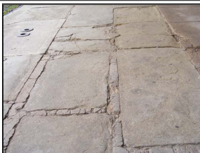
Condition 7 Extensive cracking and movement
