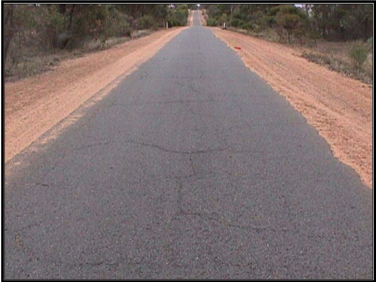
Figure 4A Bad Cracking but not a pavement problem
